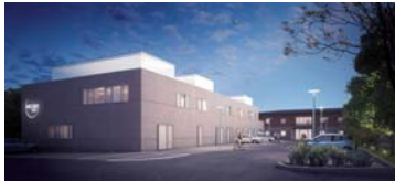
3000 m2 Offices and Workshop dedicated to Space
